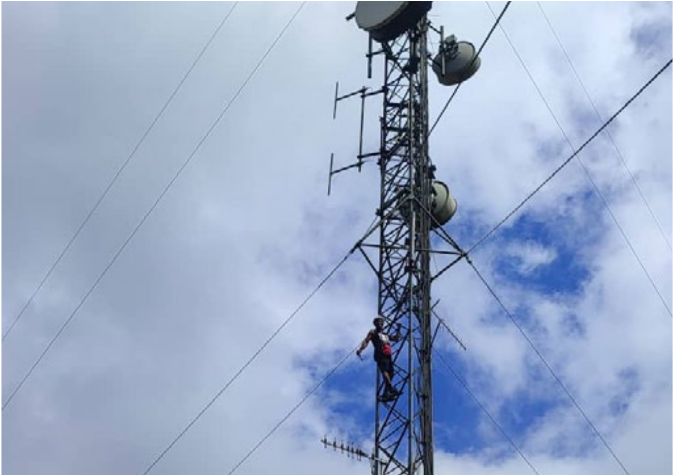
Figure 10.10 Typical FM dipole antenna sets deployed for some community and national licensed FM radios at an altitude of 1,351 metres
